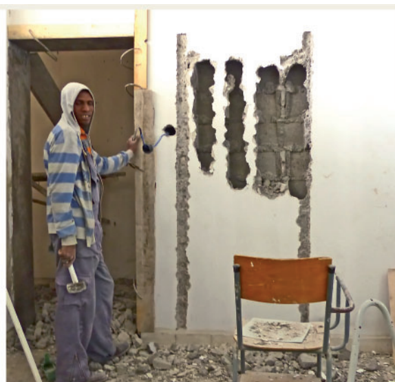
Construction of door to the cleaning room
