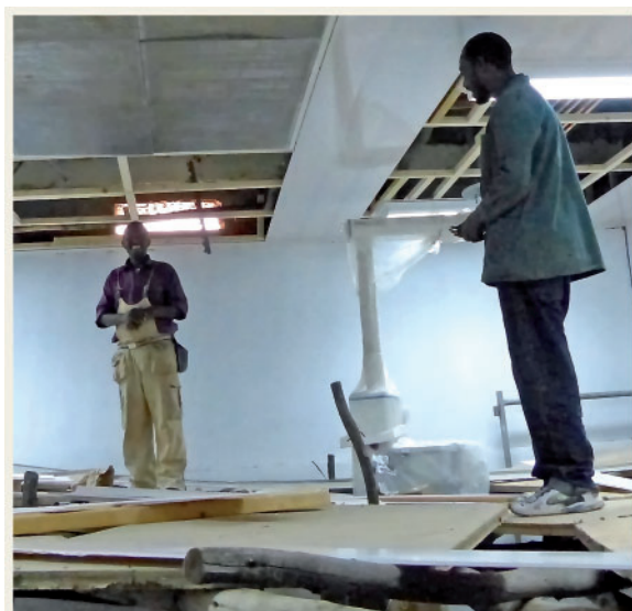
Installing ceiling of the intervention room
