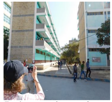
Fig. 3: no access because of electric cable and high pavement
